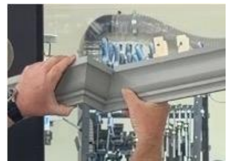
Figure 18 Short pieces coped between inside and outside corners.
